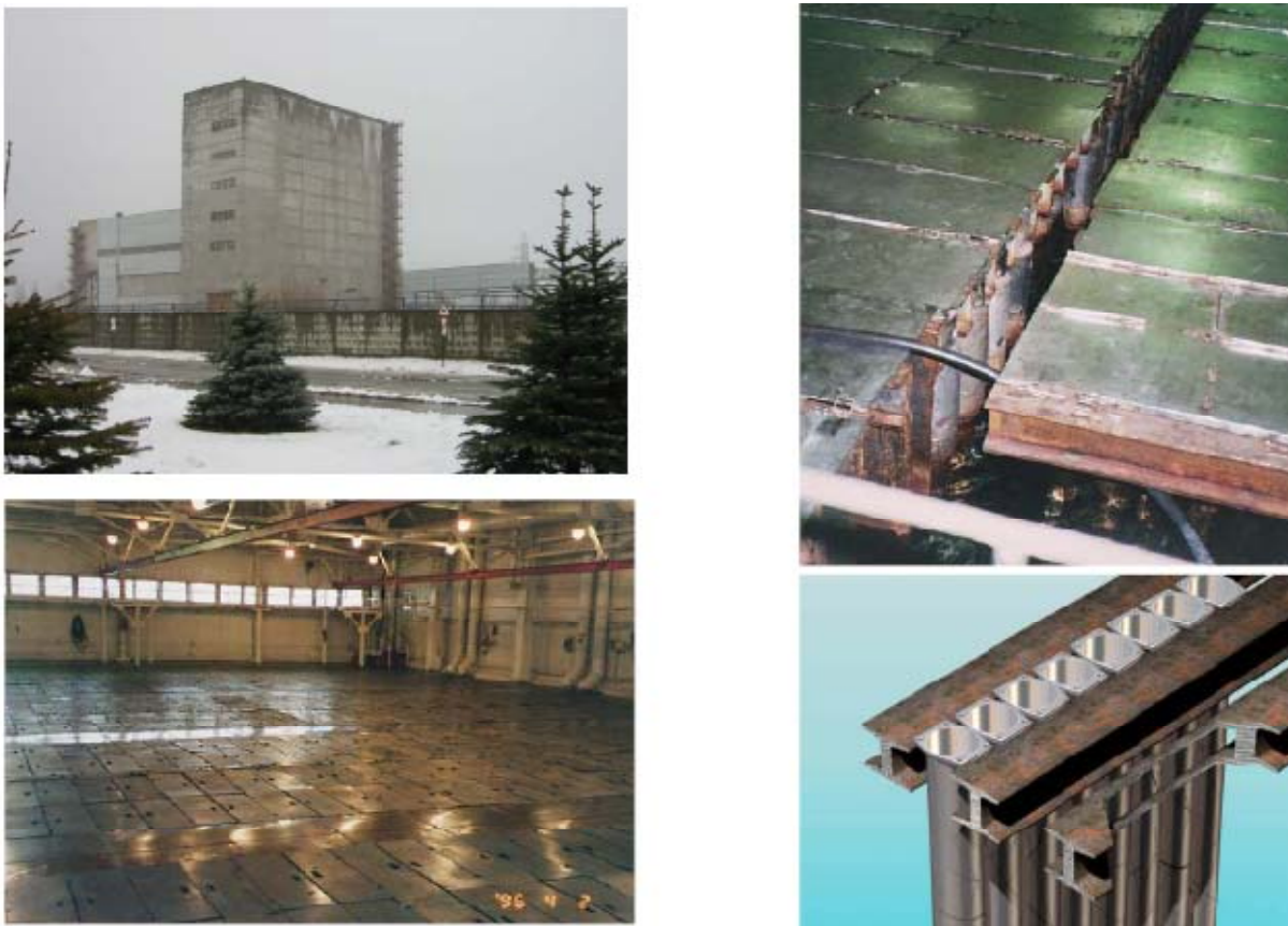
Figure 1: View of the ISF-1 from outside and the storage area (left) and details of the storage racks and cartridges (right)
