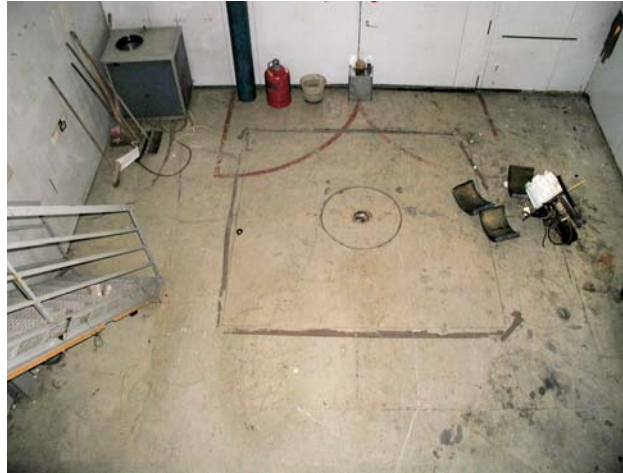
Figure 2 View into the reactor hall of the TRIGA HD I after realization of the safe enclosure by sealing the reactor top (square with a manhole for inspection reasons).
