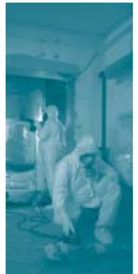
Dismantling of washer and piping.
