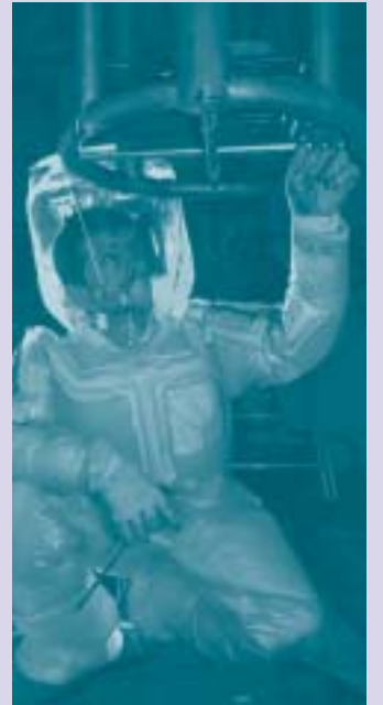
Dismantling of Brennilis NPP (France).
