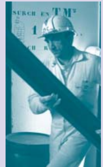
Dismantling of spent-fuel storage facility.
