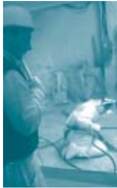
Decontamination of activated concrete parts.
