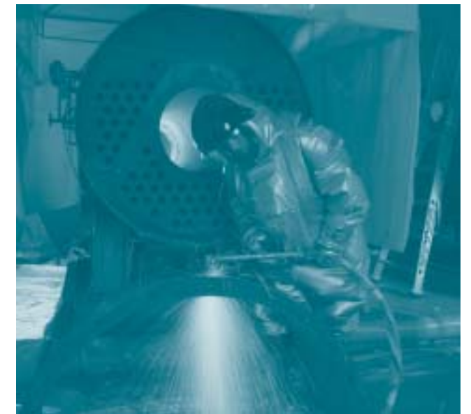
Boiler cutting performed using fire protection clothing.
