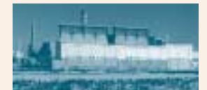
Paks Nuclear Power Plant, Hungary.
