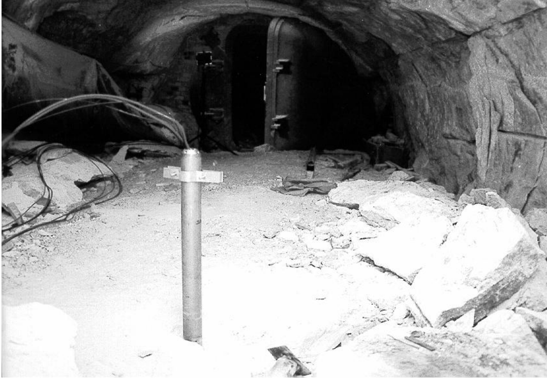
Figure 3: Open part of the drift with the packer probe installed in the borehole (in the foreground) and the door to the lined part (in the background)
